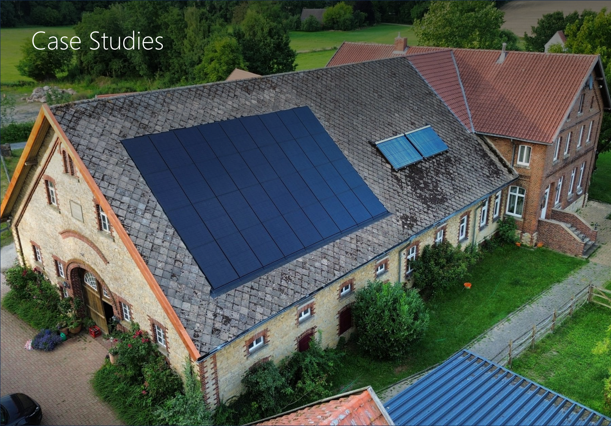
Germany Retrofit to slate roof barn
